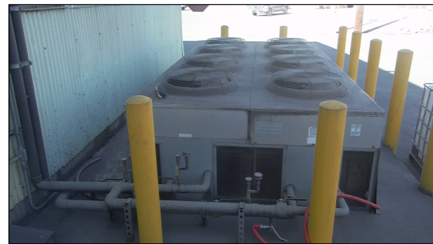
Fig. 5 Dry Air Cooler
